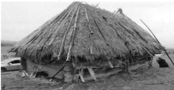
Fig. 20 The oldest way of architectural construction, Wes.Serbia
